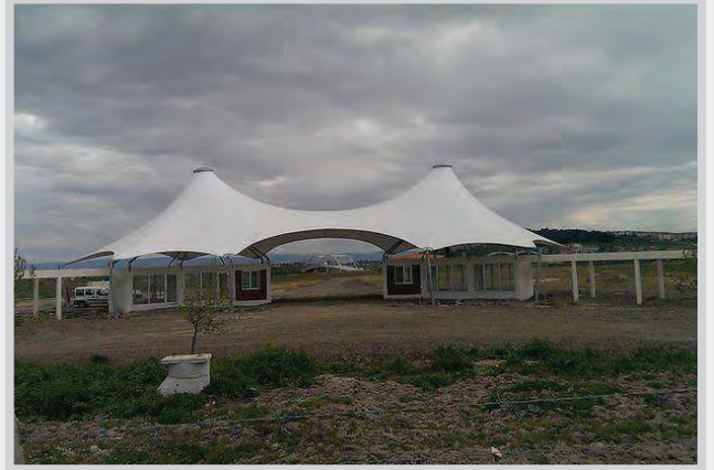
KARACABEY PARK GİRİŞ KANOPİSİ BURSA
