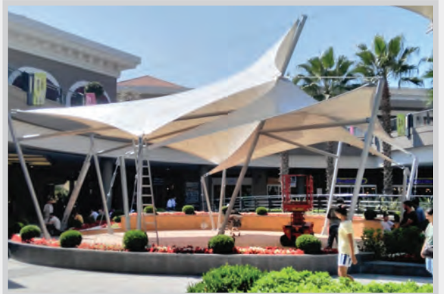
ARENA PARK OASİS CAFE İSTANBUL
